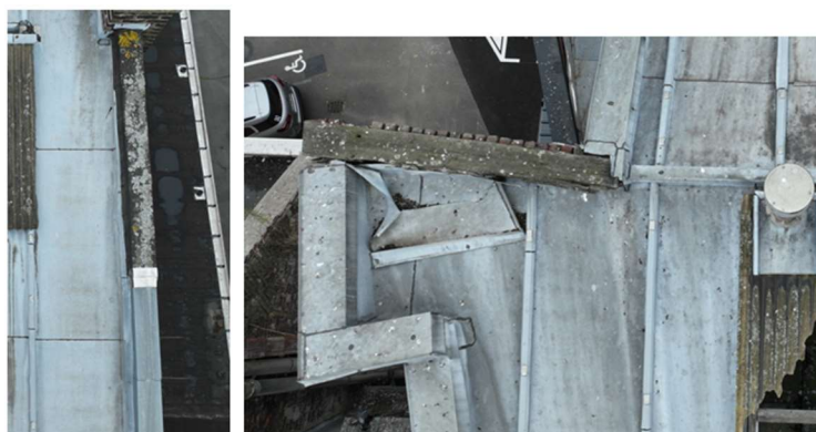
Figure 45 - Absence de couvertine
