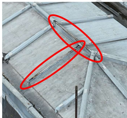
Figure 29 - Absence de couvre-joints
