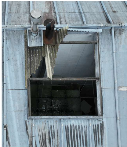
Figure 42 - Absence de couverture
